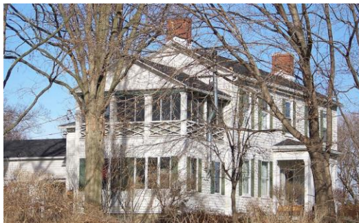
Abner Woodworth House- c. 1830 (1328 Flat St) National Register of Historic Places
