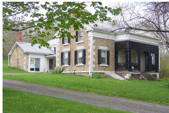
Angus family cobblestone house 1831-34 (612 Route 14) House and Barn National Register of Historic Places
