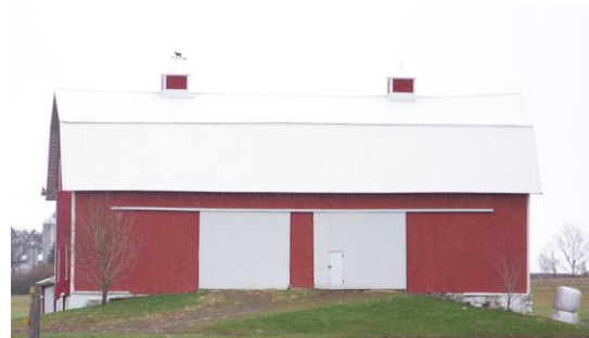
Barn with double cupolas 1880's ( 1898 E. Havens Corners Rd)
